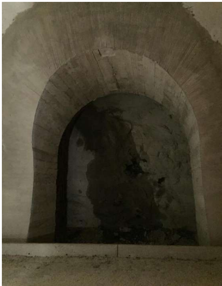
Figura 4 – Galleria Guinza – E78 – By-pass pedonale.
