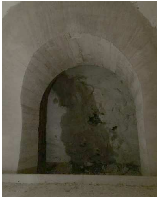
Foto 3 – Galleria Guinza - By pass pedonale
