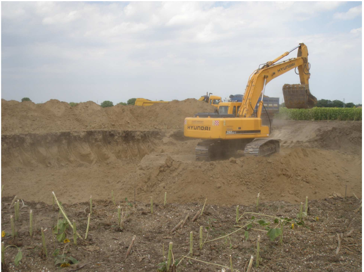
Figure 8.1: Typical excavation process
