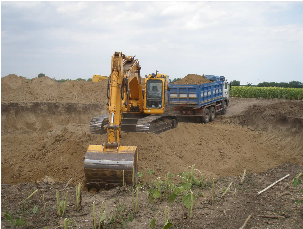
Figure 8.2: Typical excavation process
