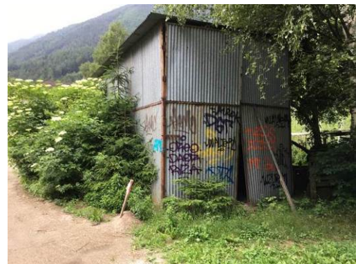
Baracca – Barackenlager “A8”
