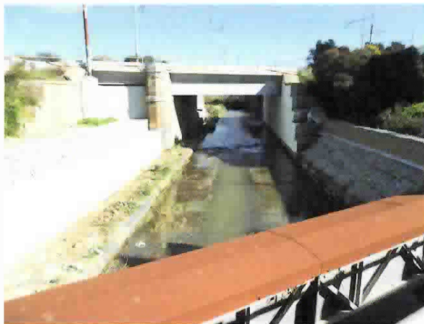
POST OPERAM – area intervento 2-3
