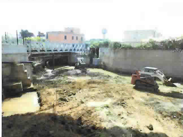
ANTE OPERAM – area intervento 4
