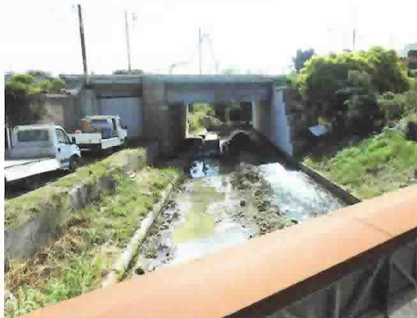
ANTE OPERAM – area intervento 2-3
