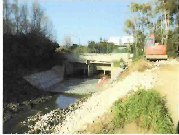
POST OPERAM – area intervento 15
