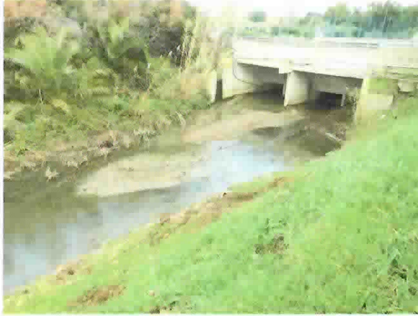
ANTE OPERAM – area intervento 15
