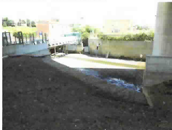
POST OPERAM – area intervento 4
