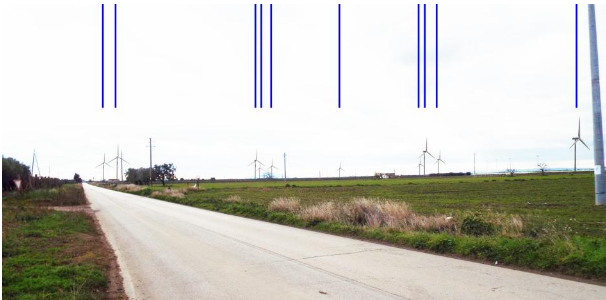
Vista 2A_1 post operam
