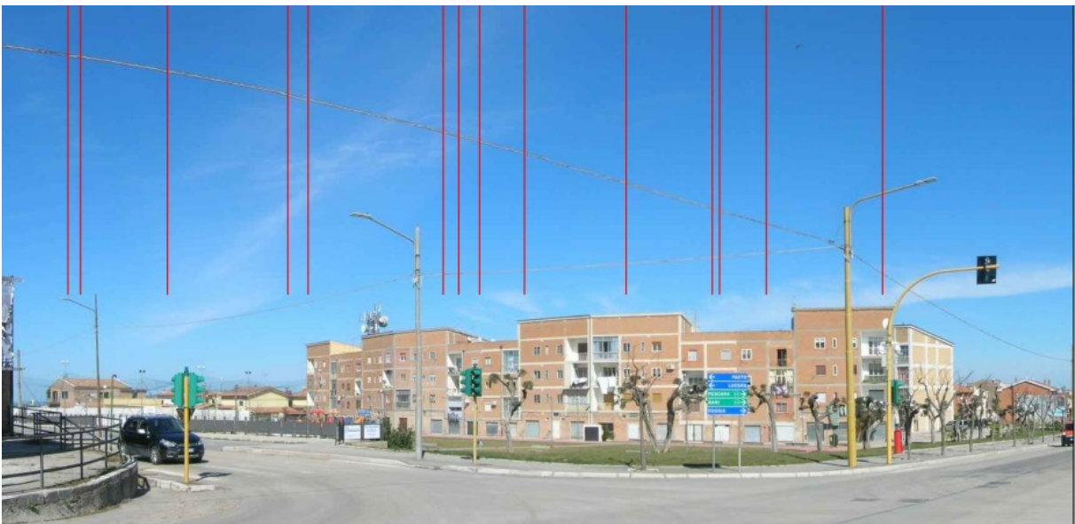
Vista 9_2 post operam
