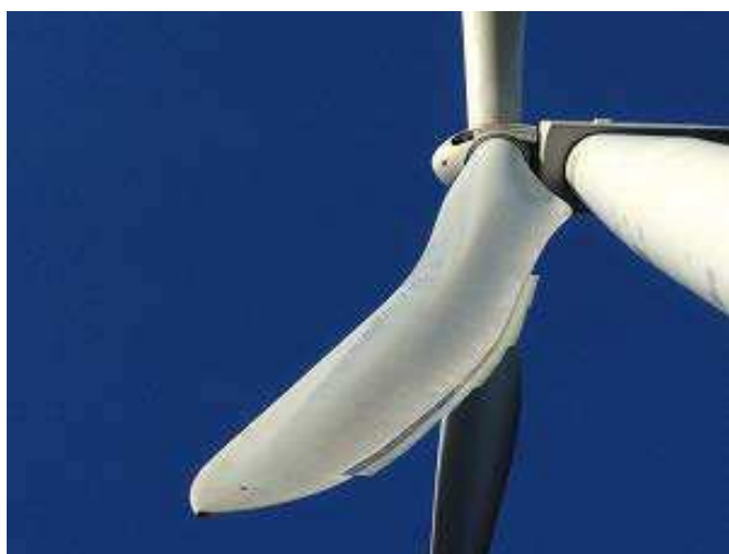
Fig. 1: LNTEs at the wind turbine rotor blade
