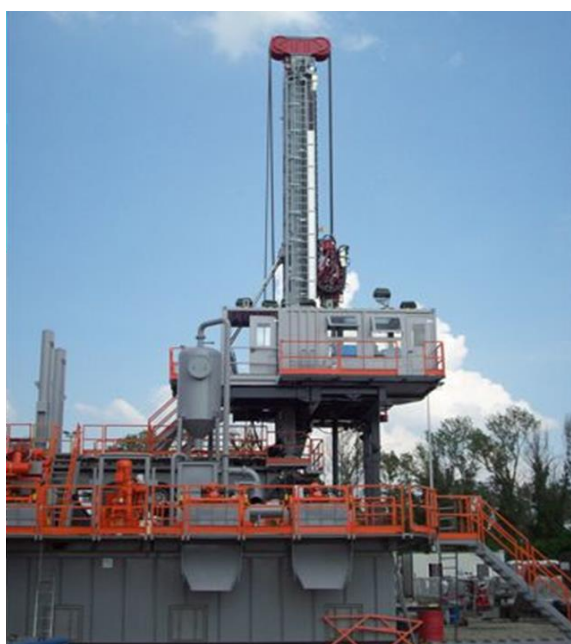
Figura 5.d: Impianto Drillmec HH-200MM
