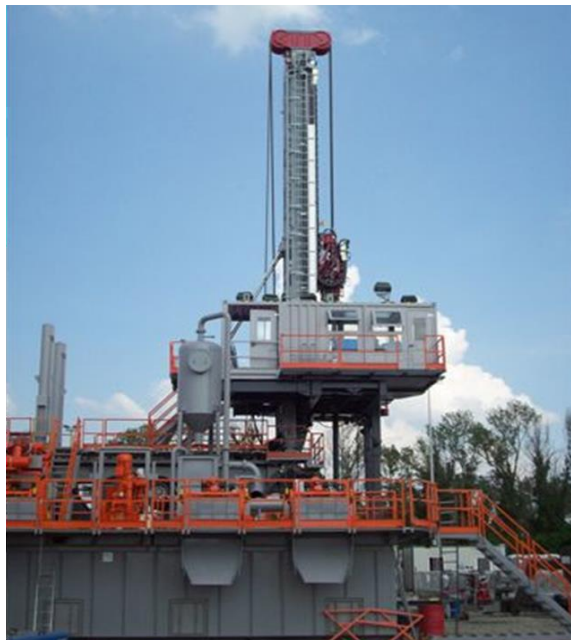
Figura 4.c: Impianto Drillmec HH-200MM
