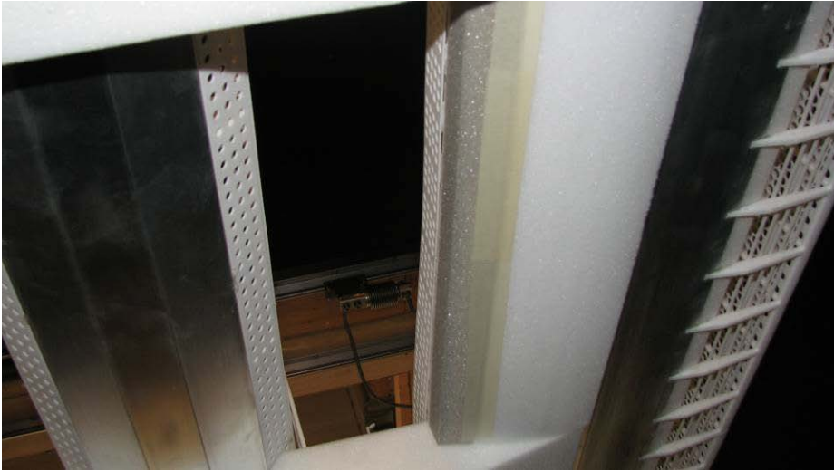
Figure 3.5. Photograph of sharp edge configuration – road deck girder.
