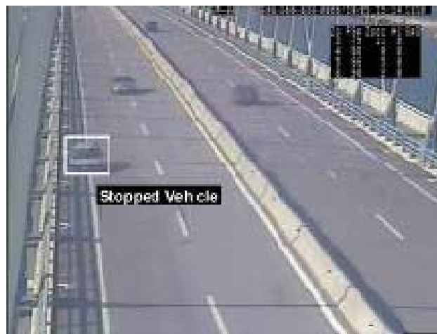
Figure 5.8.8: Example showing an AID system detecting a stopped vehicle on a bridge
