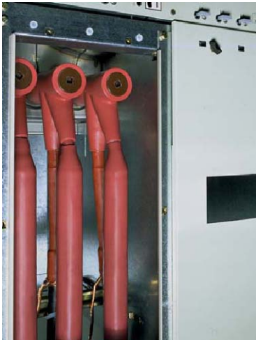
Fig. 5.12.9 Switchgear with arrester Raychem, or similar
