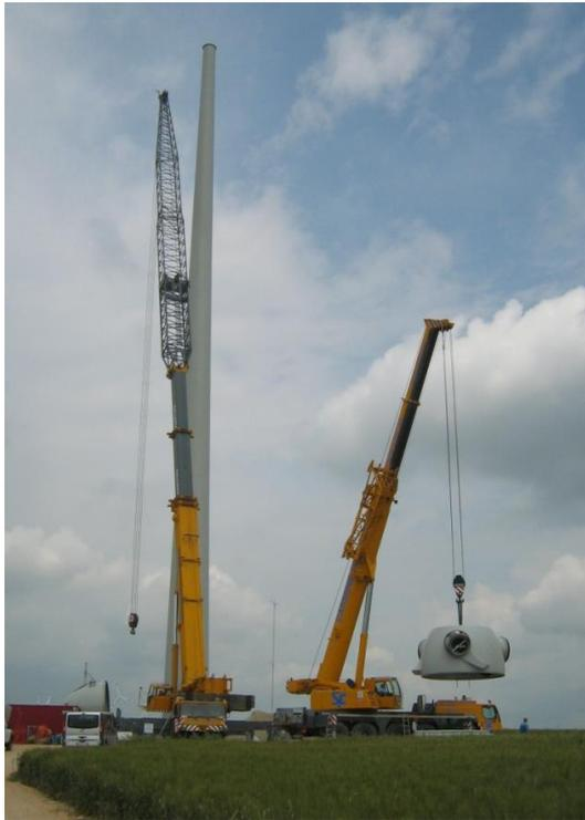
**Figura 3:** smontaggio navicella
