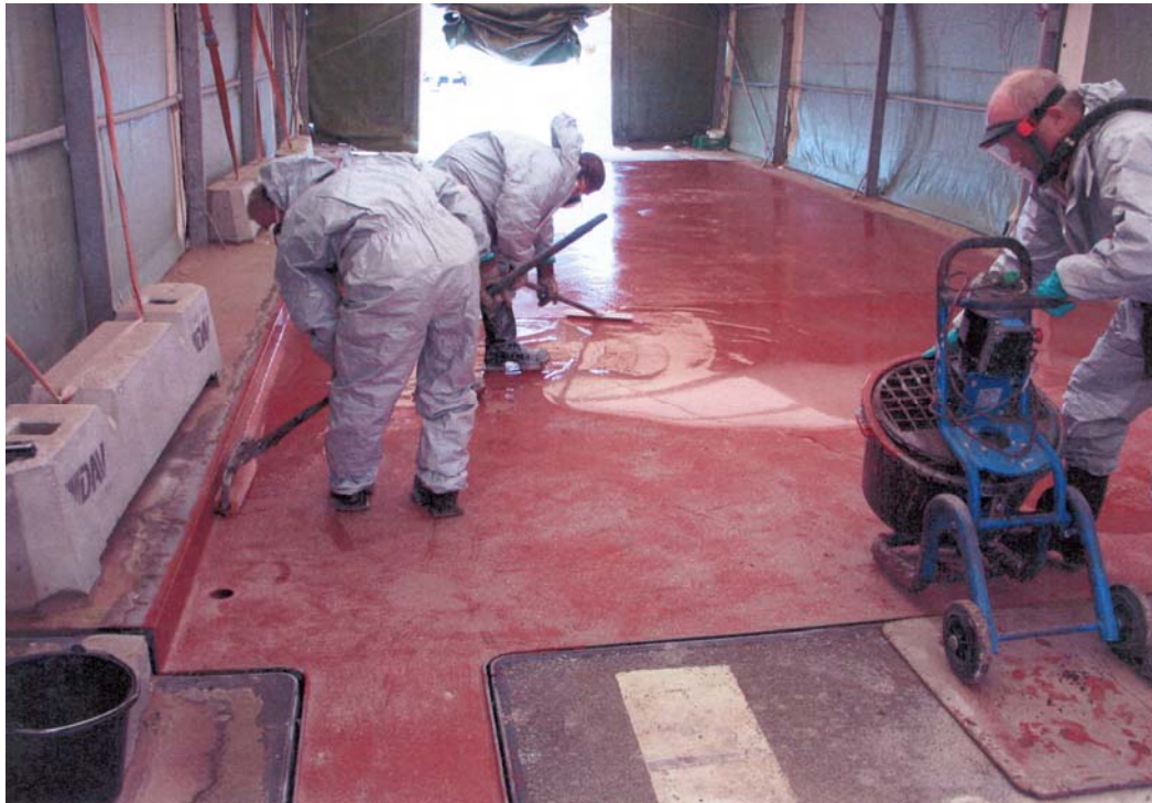
Figure 3 Application of the membrane by roller
