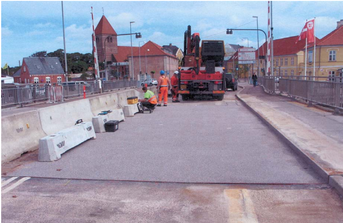
Figure 4 Completed thin surfacing on small bridge in Denmark, 2010
