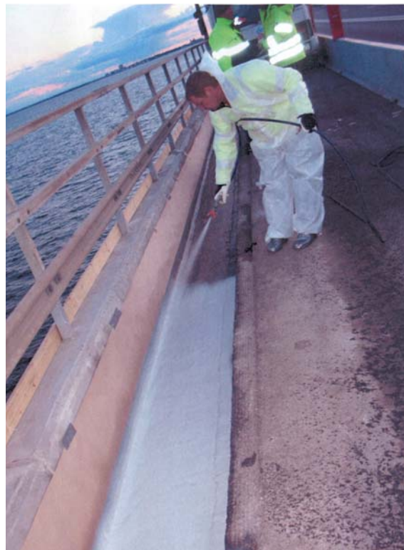
Figure 2 Application of primer by airless spray
