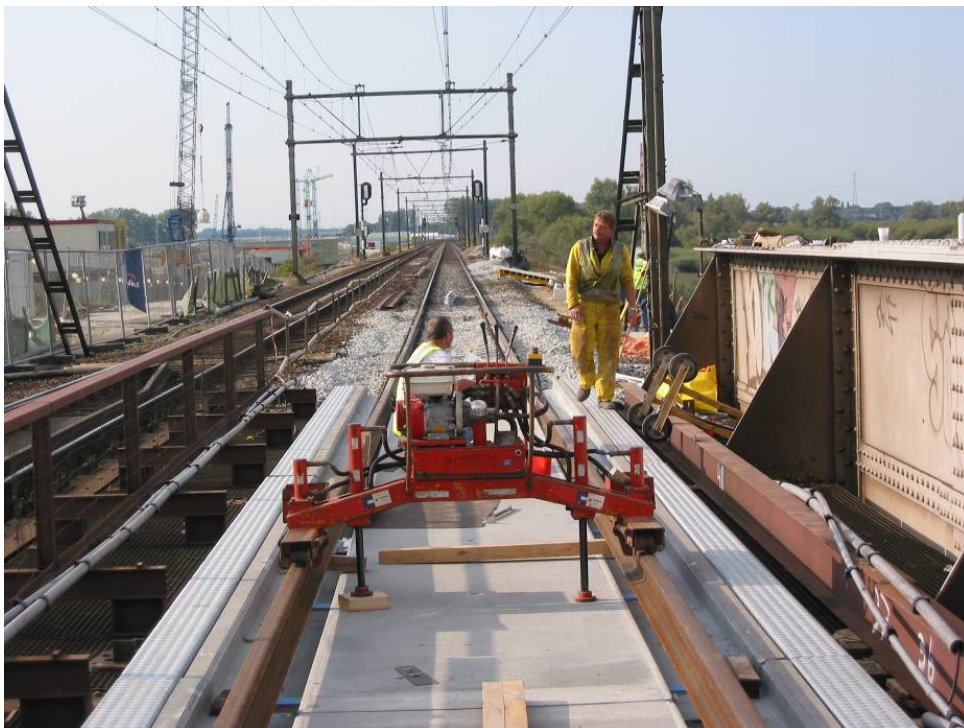
Figure 13 Installation of rails using top-down procedure
