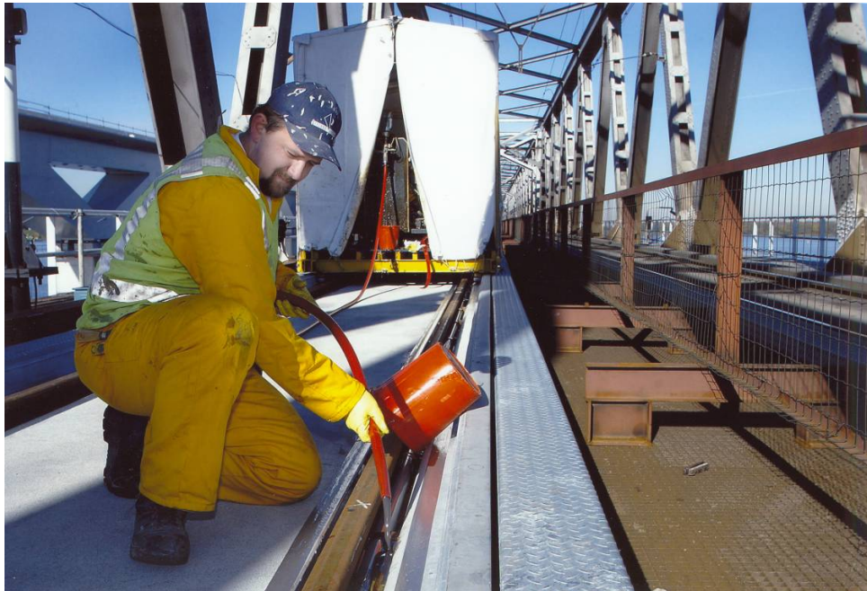
Figure 14 Pouring of Edilon Corkelast
