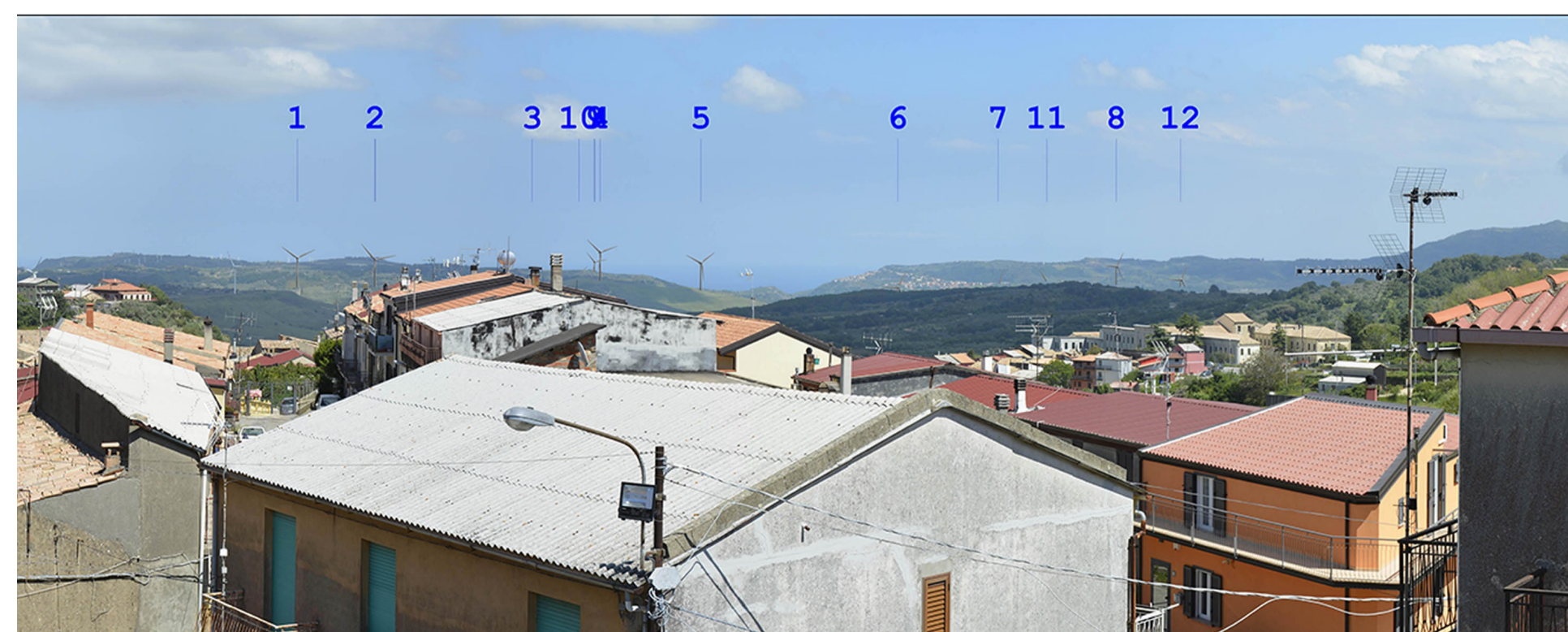
Vista post operam
