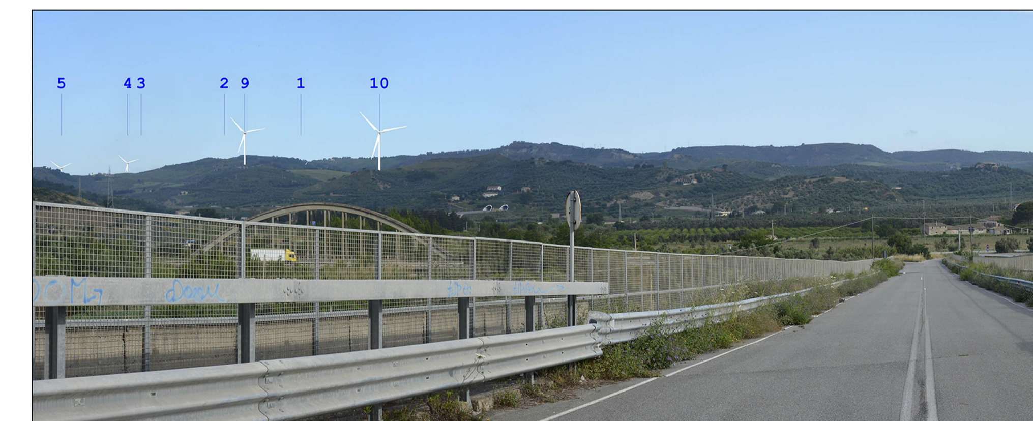
Vista post operam
