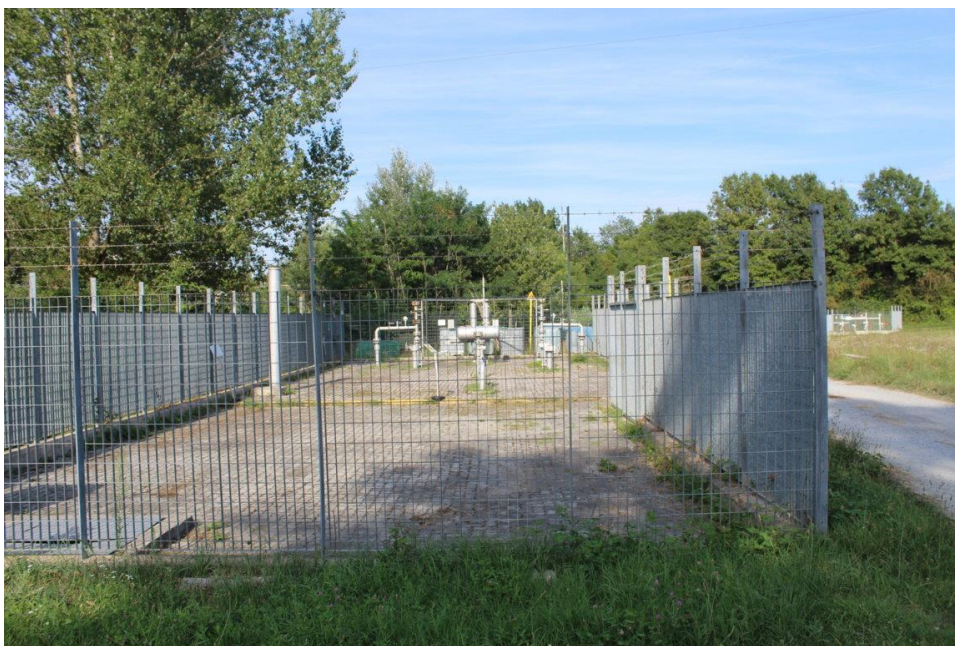
RP-31 – AREA INTERVENTO 5 – RIF. PIDI 4500240/20.1
