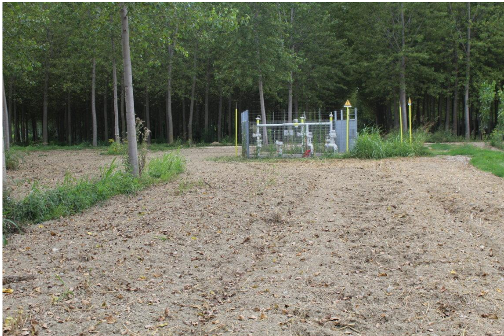
RP-20 – AREA INTERVENTO 3 – RIF. PIDI 4500240/5.0.1
