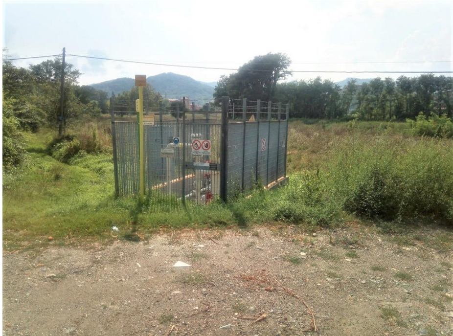
RL-2 – AREA INTERVENTO 6 – RIF. PIDI 4500240/33
