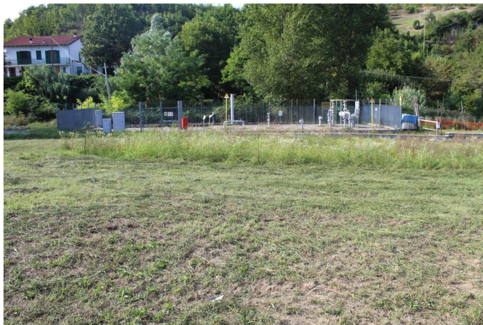
RP-30 – AREA LATERALE INTERVENTO 5 – RIF. PIDI 4500240/20.1
