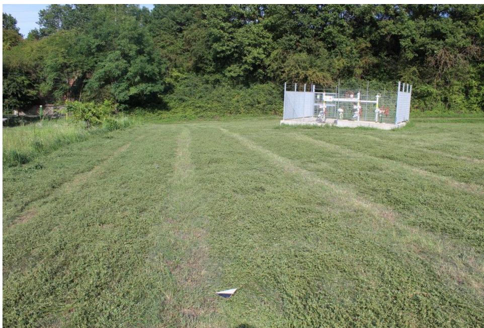
RP-29 – AREA INTERVENTO 5 – RIF. PIDI 4500240/20.1
