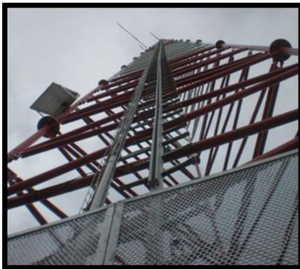
Figure 6. Fall arrest system
