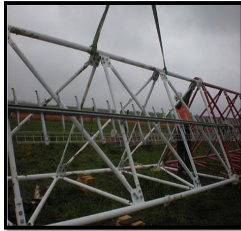
Figure 2. Met Mast Structure
