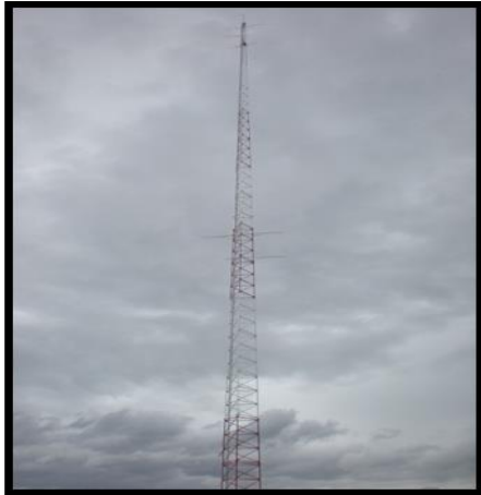
Figure 1. Met Mast Structure
