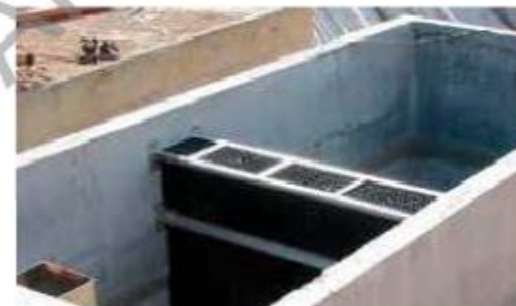
Layout con filtro verticale. Vertical filters installation.
