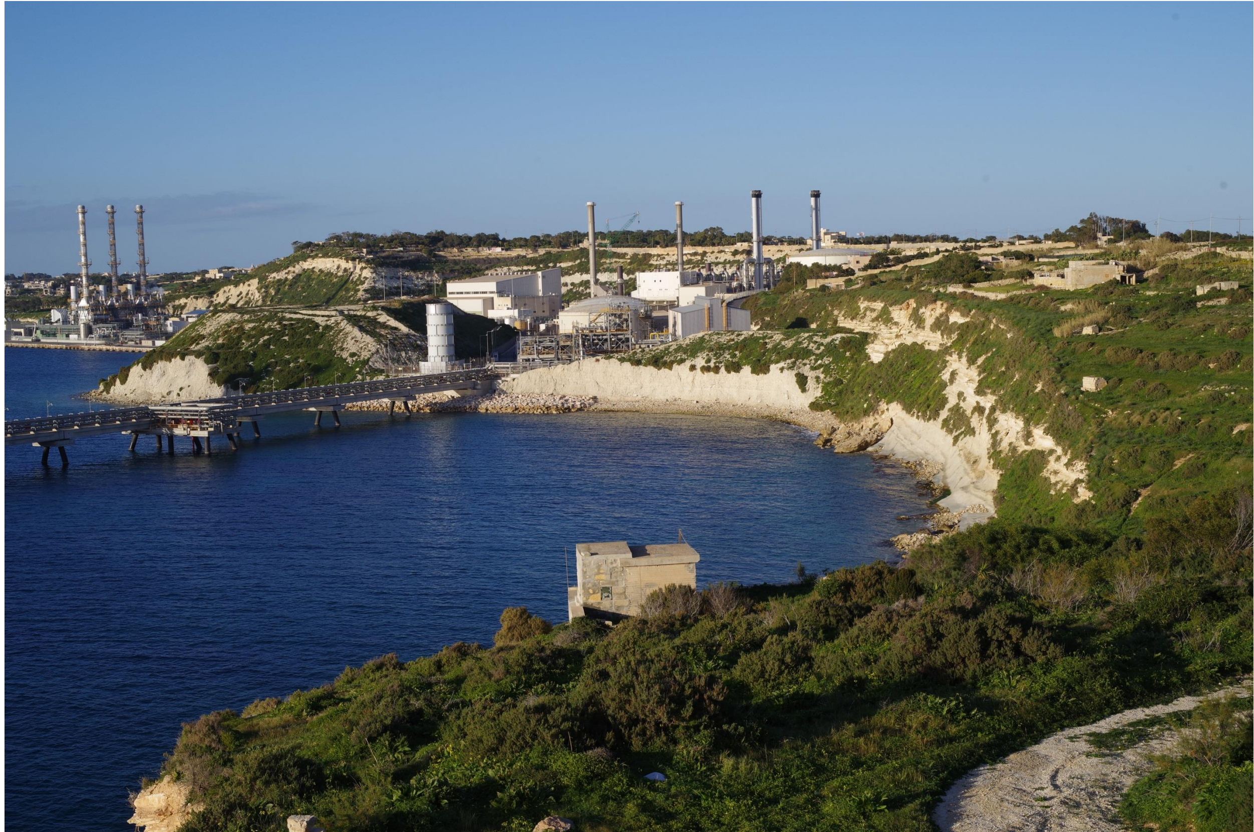
Figure 4: Viewpoint (VP 1) from carpark overlooking Delimara Power Station
