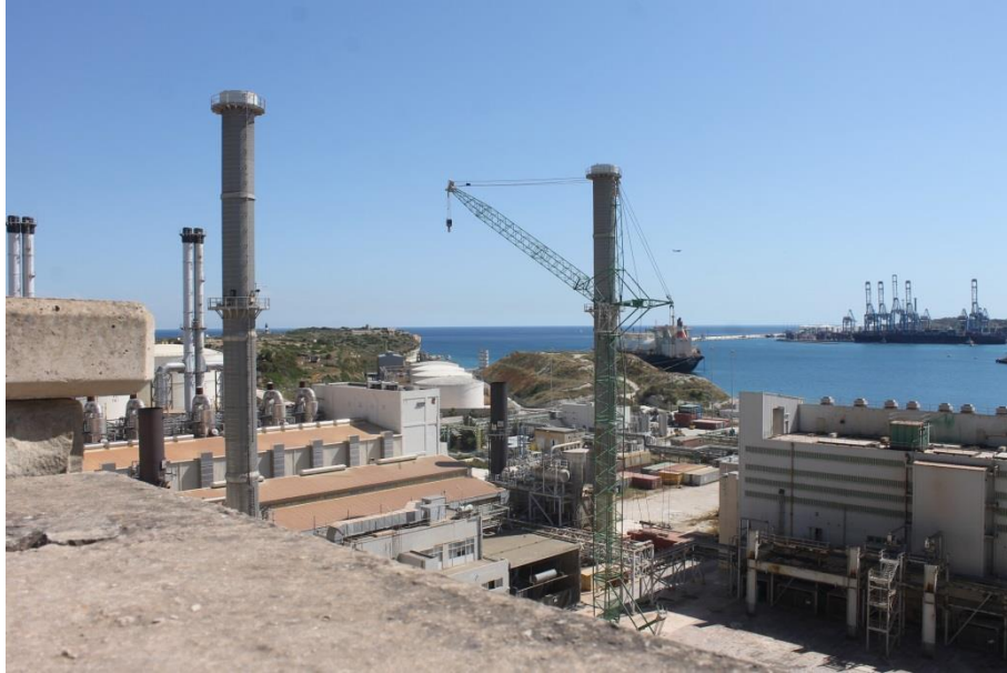
Figure 11: Delimara Power station and FSU in the distance
