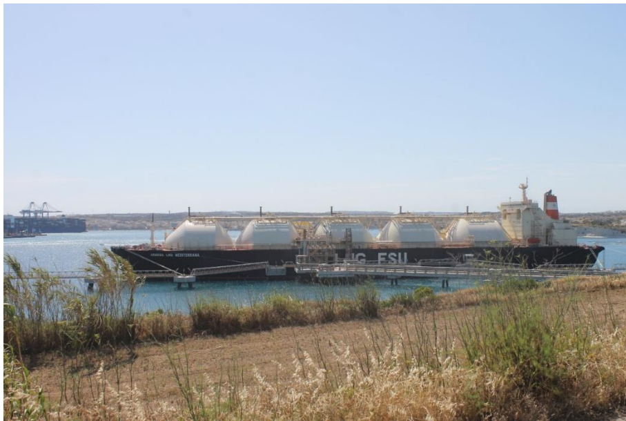
Figure 12: Floating storage unit (FSU) and jetty linked to the Delimara Power Station
