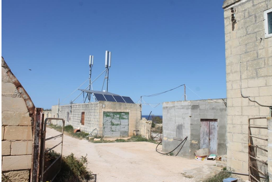
Figure 11: Antennae in broadcasting station
