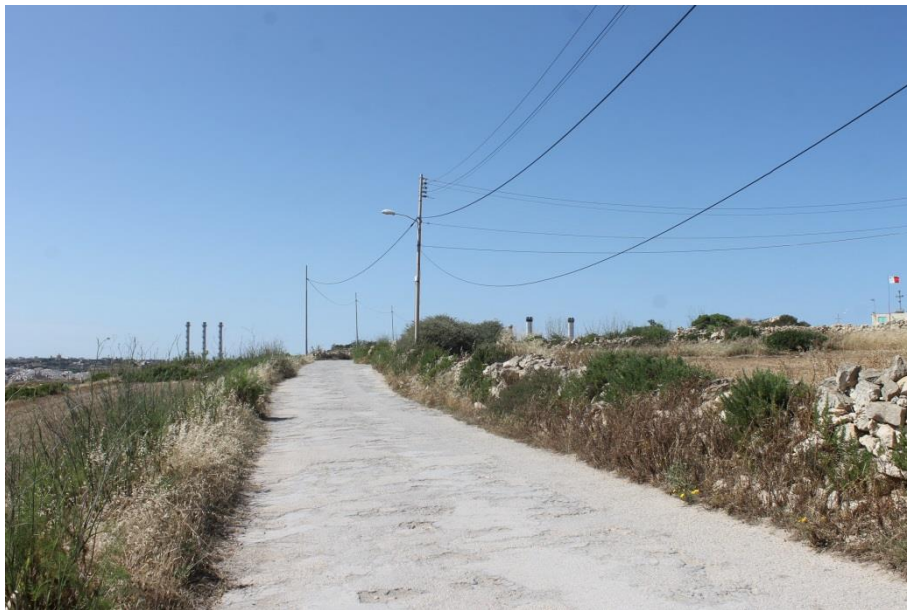
Figure 10: Street lighting and aerial cables
