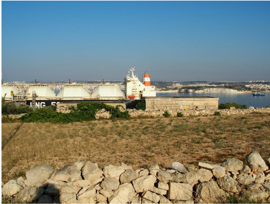
Figure 37: Photo 10 - Secondary use structure; looking West.
