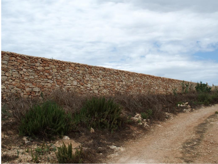
Figure 35: PHOTO 8 - Farmhouse wall: looking N East.
