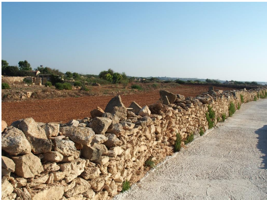
Figure 32: PHOTO 5 - Dry-Stone walls; looking North.
