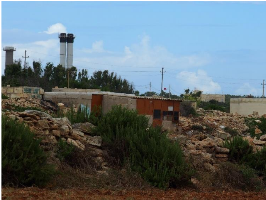
Figure 40: PHOTO 13 - Non-residential structure; looking N West.
