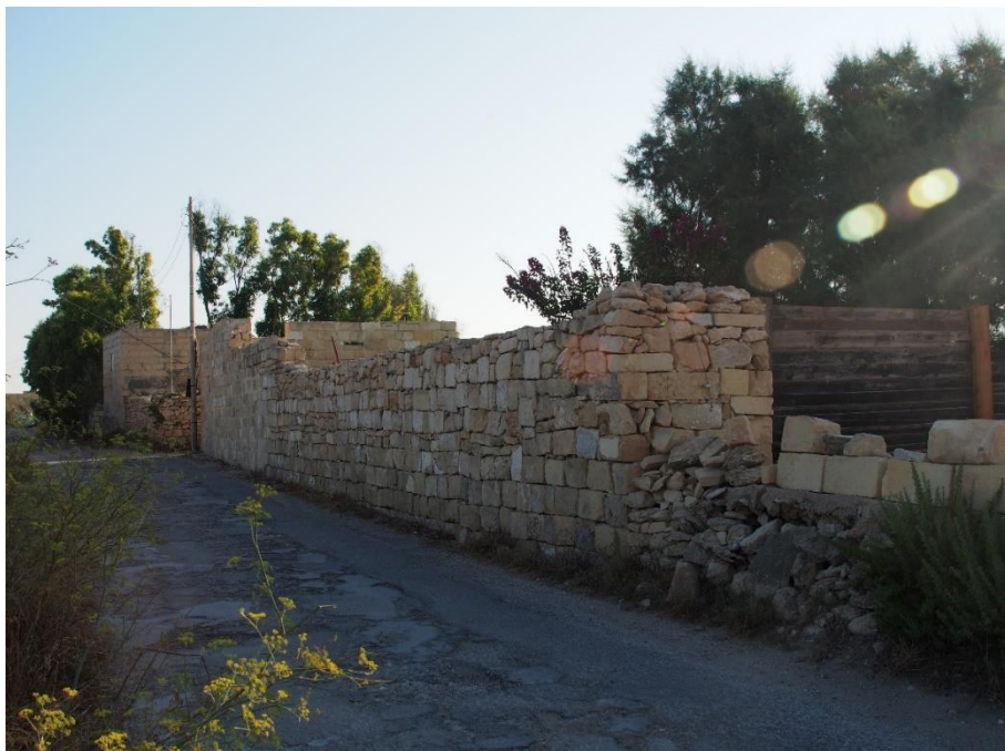
Figure 34: PHOTO 7 - Dry-Stone walls; looking North.
