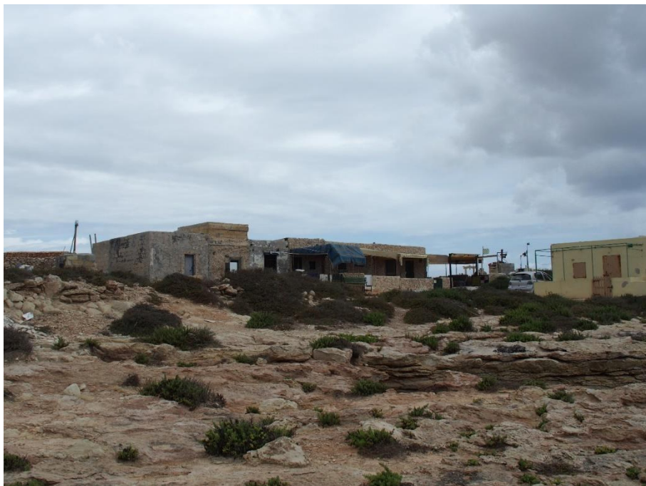
Figure 42: PHOTO 15 – Residential unit; Looking West.
