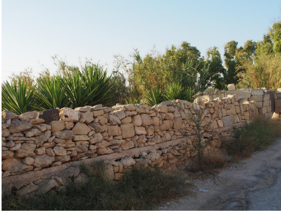
Figure 33: PHOTO 6 - Random rubble stone wall with concrete intrusions; looking South.
