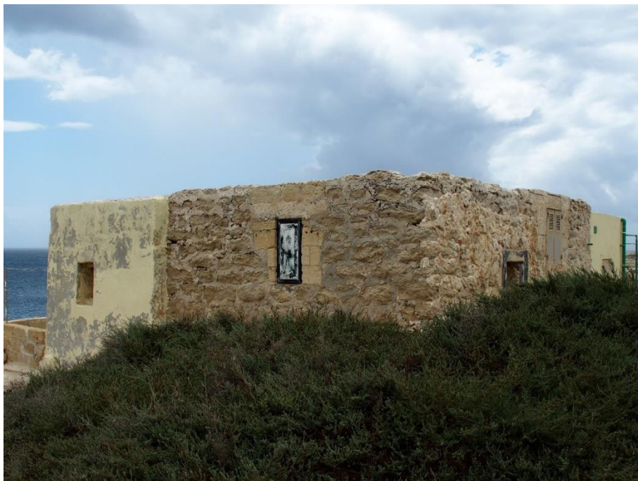
Figure 38: PHOTO 11 - Secondary use structure; looking South.
