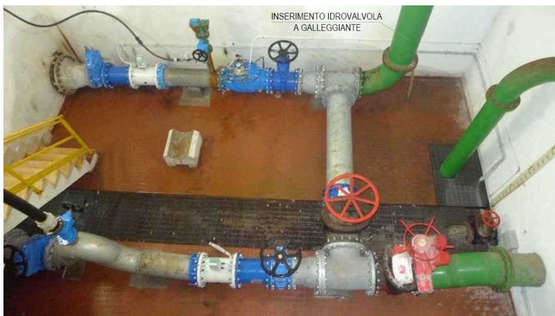
Figura 4.3 – Camera valvole serbatoio Succoronis
