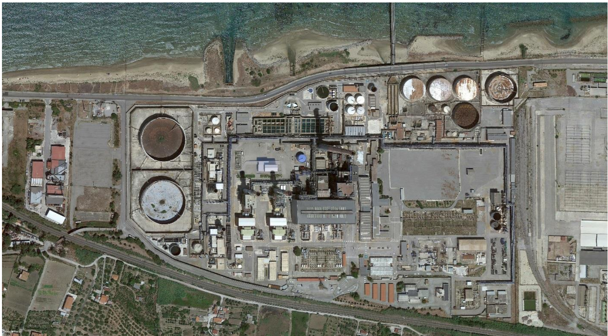
Figura 4.7.14: Vista zenitale – Post operam
