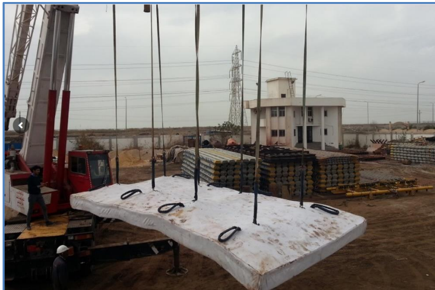
Figure 4.30 – Cable Crossing – Typical Bitumen Mattresses
