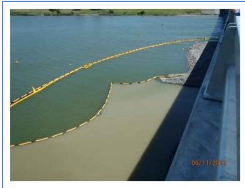
Figure 4.27 – Post-trenching Filter Barrier Example
