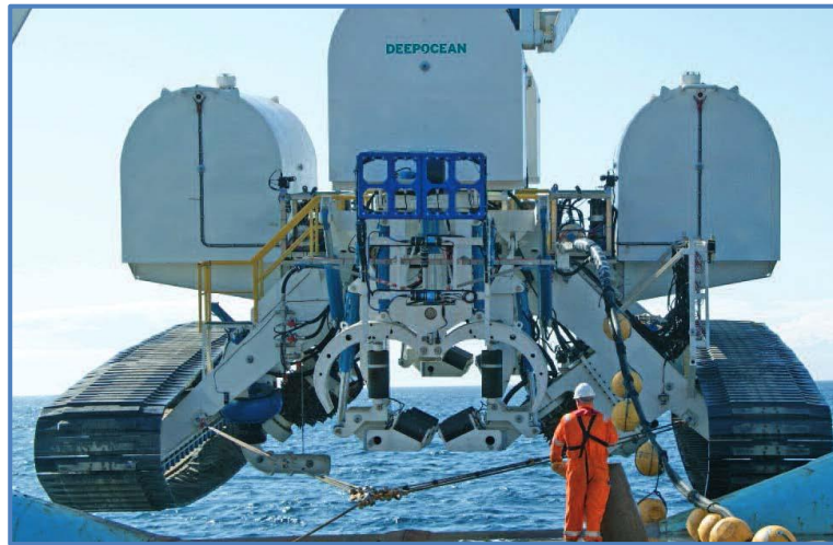
Figure 4.21 – Post-trenching Works – Example of Suction Cutter Equipment
