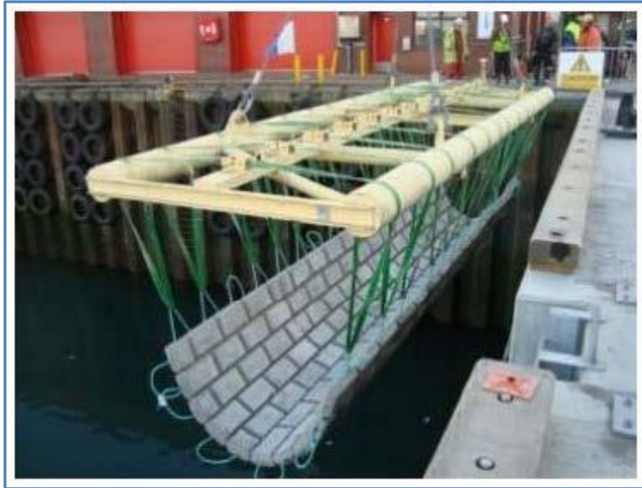
Figure 4.29 – Cable Crossing – Typical Concrete Mattresses
