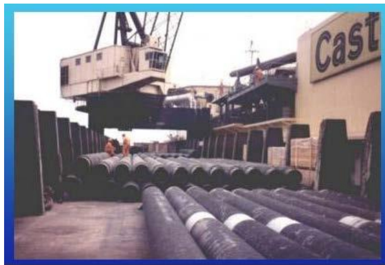
Figure 4.9 – S-lay Vessel – Typical Pipe Joint Stacking Area
