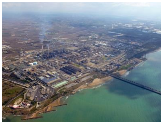
Figure 34: Industrial area of Gela
