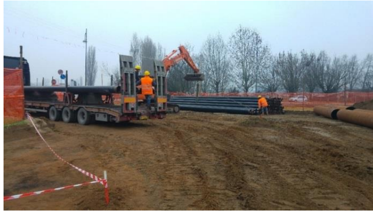
Figure 3: Example of Temporary Working/Storage Area
