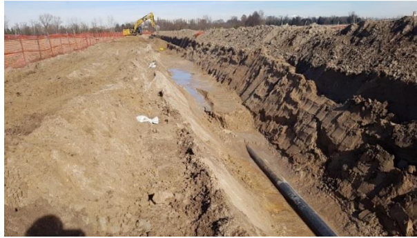
Figure 6: Backfilling of the pipeline
