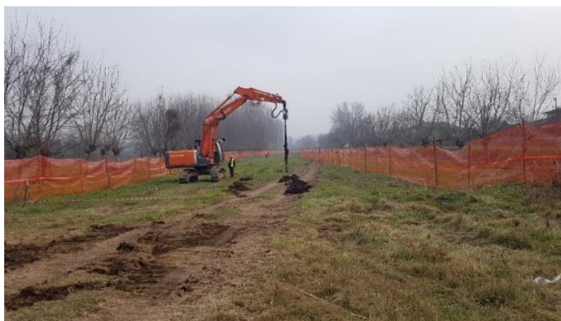
Figure 2: Example of Demining activity along the ROW
