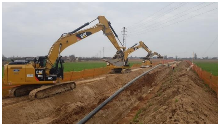
Figure 5: Laying of the pipeline string
