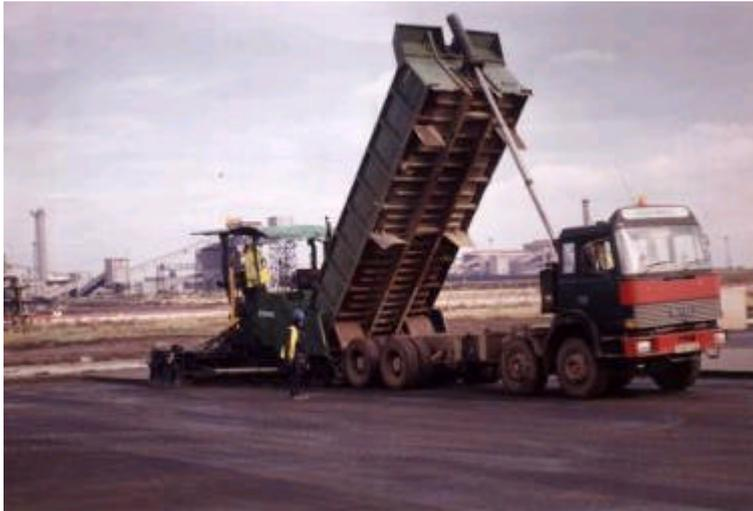
**Figure 2 - Paving PFA modified CBM 4 roadbase**
