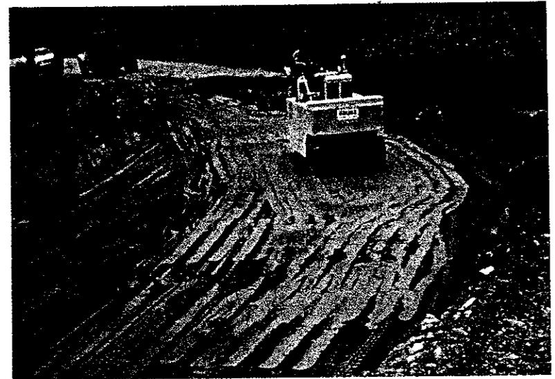
Figure 21. Highway embankment with fly ash structural fill.
