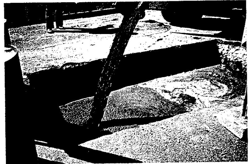
Figure 14. Flowable fill used as backfill material for a utility trench allows rapid return of traffic to the roadway.
