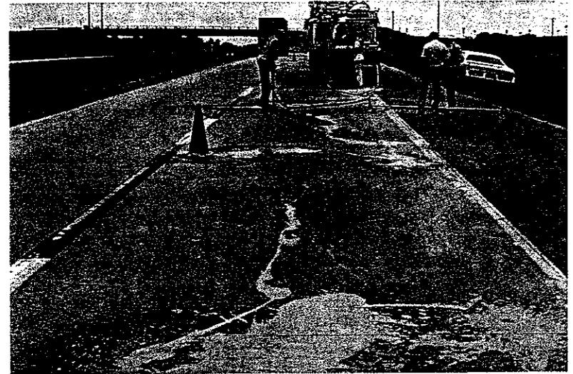
Figure 19. Fly ash grouts for pavement subsealing.
