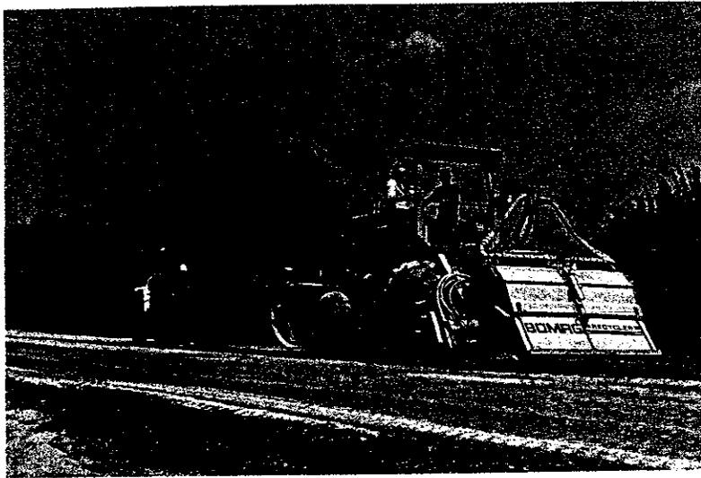
Figure 11. In-place mixing of fly ash-stabilized roadbase.
