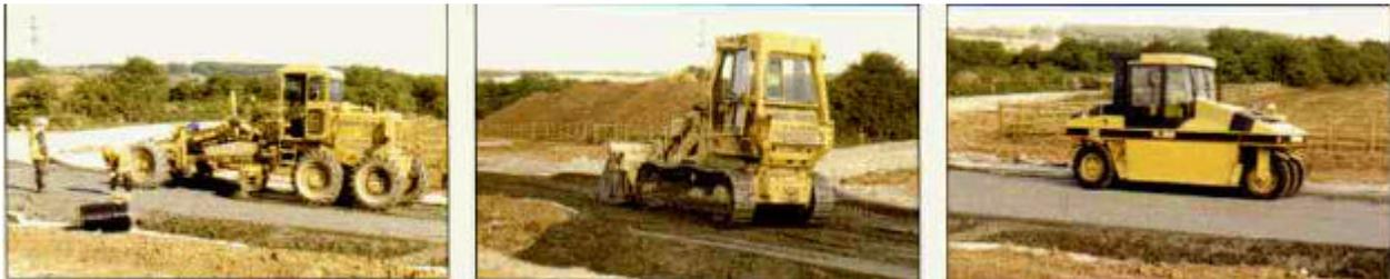
Gotham by-pass, Notts. Levelling / Laying CFA. Gotham by-pass, Notts. Levelling / Laying CFA. Gotham by-pass, Notts. compacting CFA.
