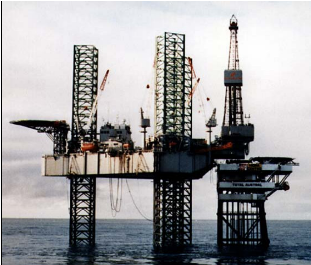
Figura 3-5: impianto Jack-Up Drilling Unit (tipo "GSF Key Manhattan")
