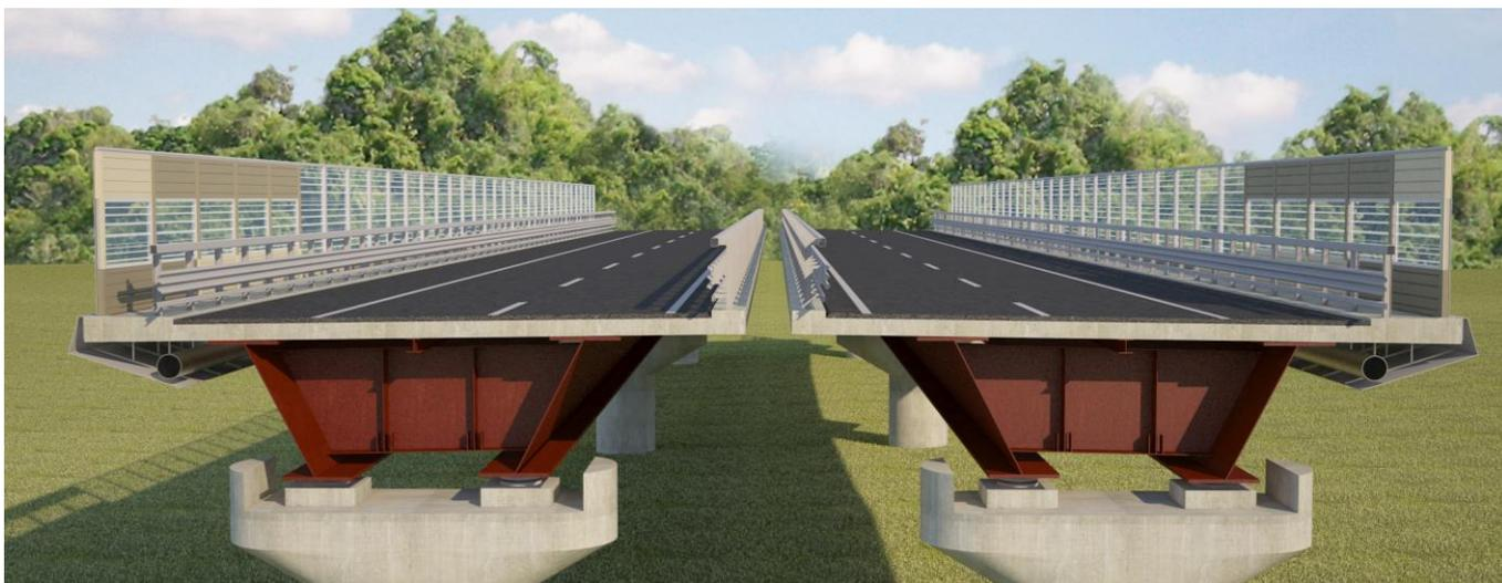
**FIGURA 4-28 – SPACCATO DI VIADOTTO AD IMPALCATO METALLICO IN ACCIAIO COR-TEN**
