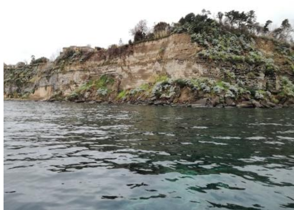
Vista costone in dissesto
