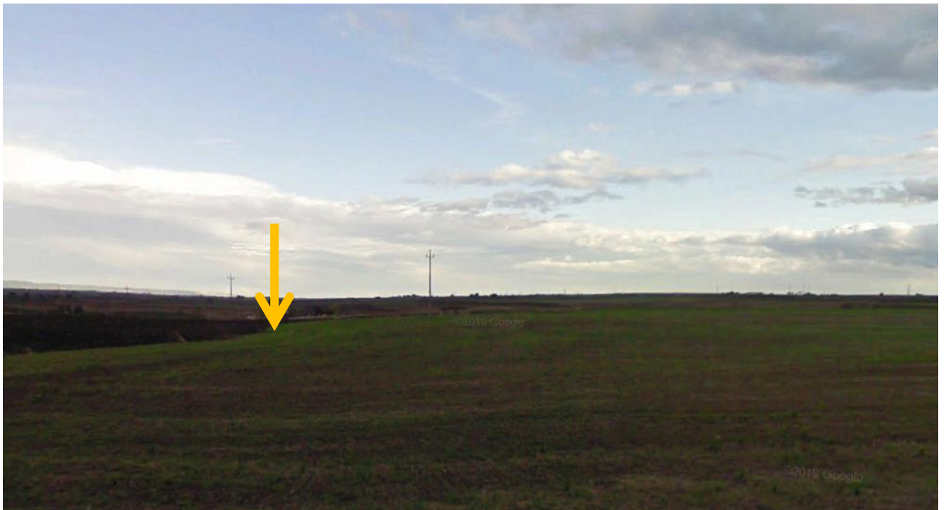
Figura 2-9: Vista turbina WTG 6
