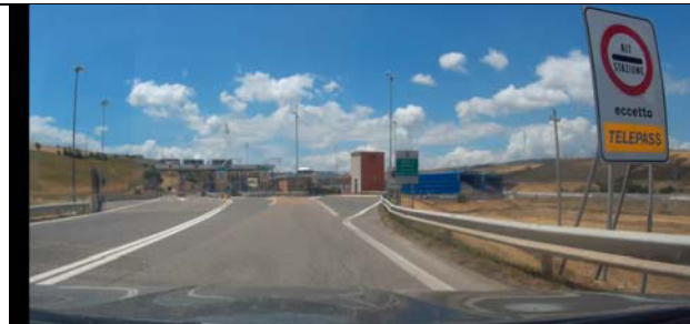
41°04'55.8"N 15°21'57.1"E, Highway exit
