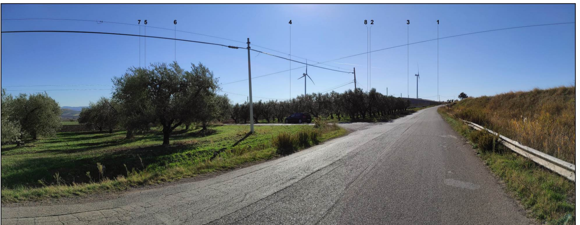
Vista 18_2 post operam
