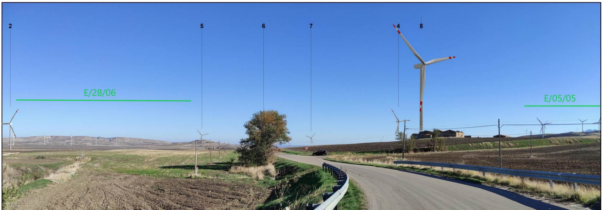
Vista V1_3a post operam
