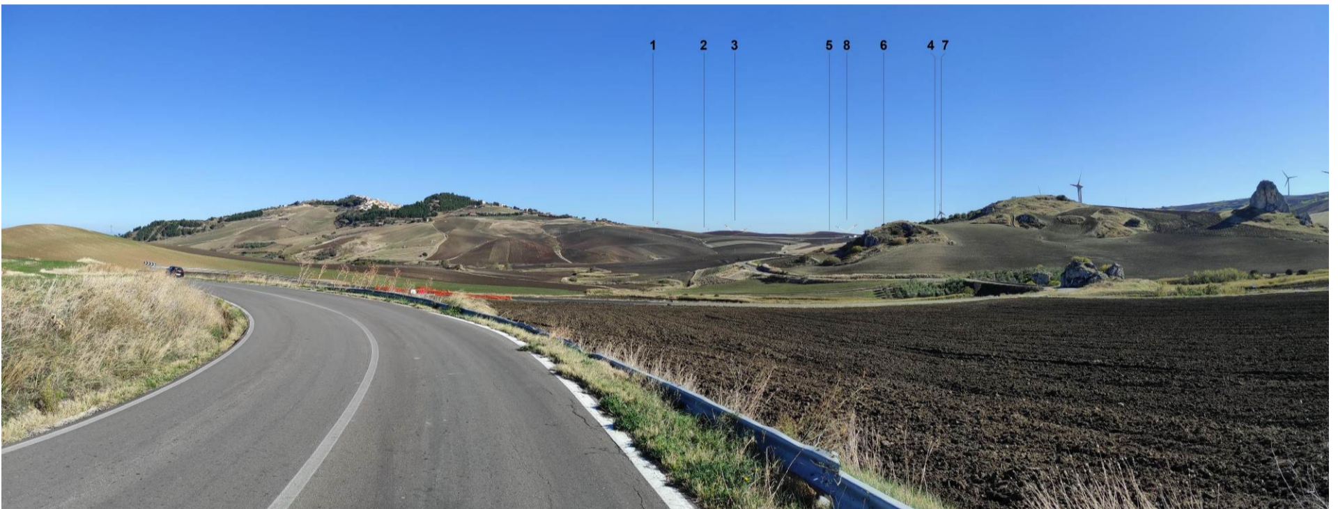
Vista 5_2 post operam
