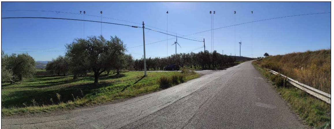
Vista 18_2 post operam
