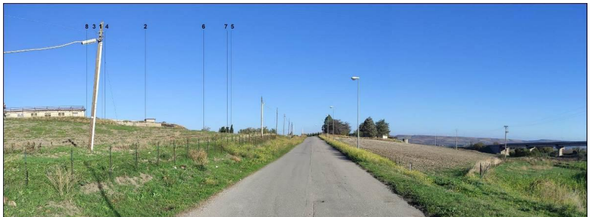
Vista 12 post operam
