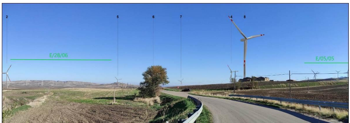
Vista V1_3a post operam
