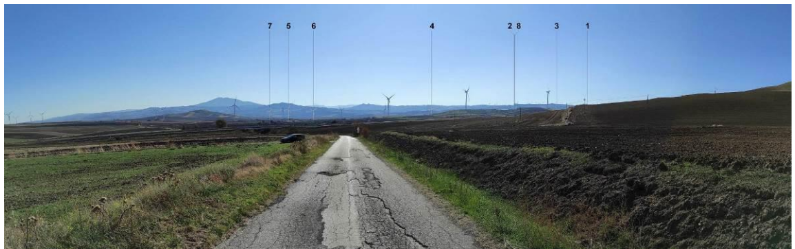
Vista 18_1 post operam
