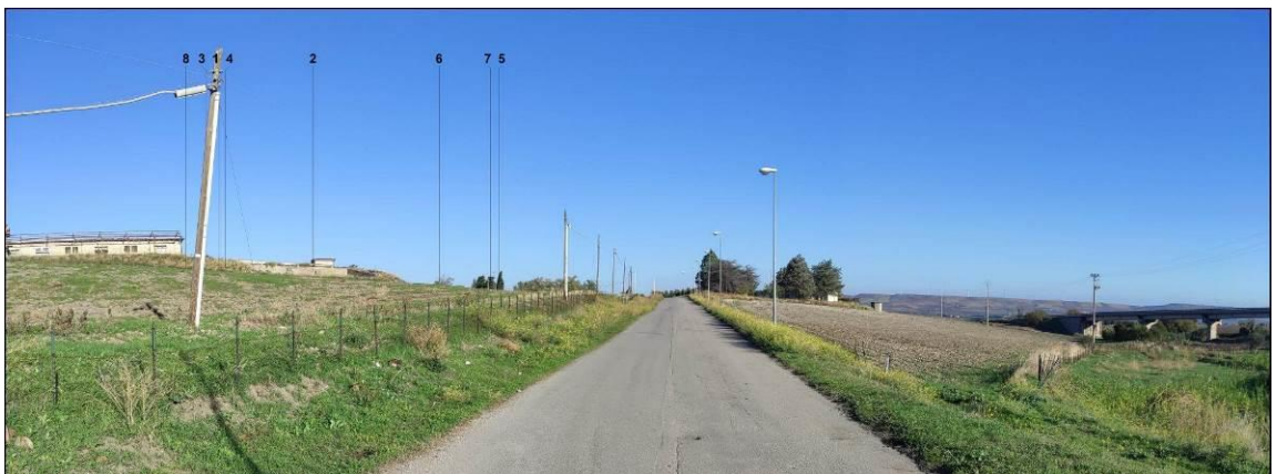
Vista 12 post operam
