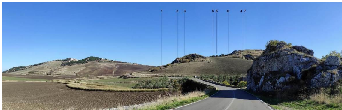
Vista 5_1 post operam
