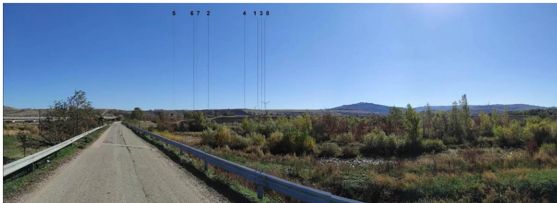
Vista 23 post operam
