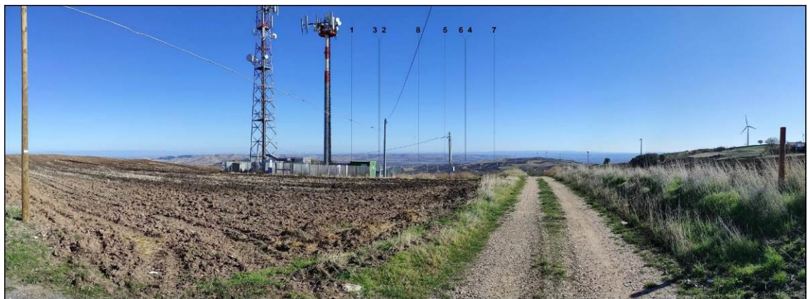
Vista 8 post operam
