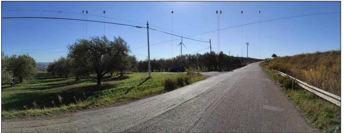
Vista 18_2 post operam
