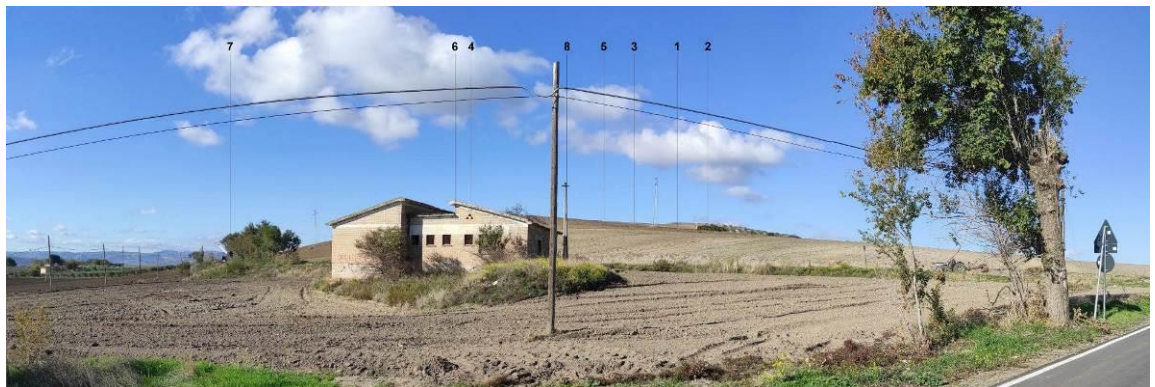
Vista 14 post operam
