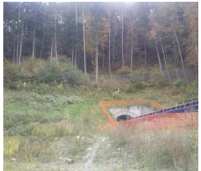
Portal Aicha-Hinterrigger Portale Aica-Hinterrigger
