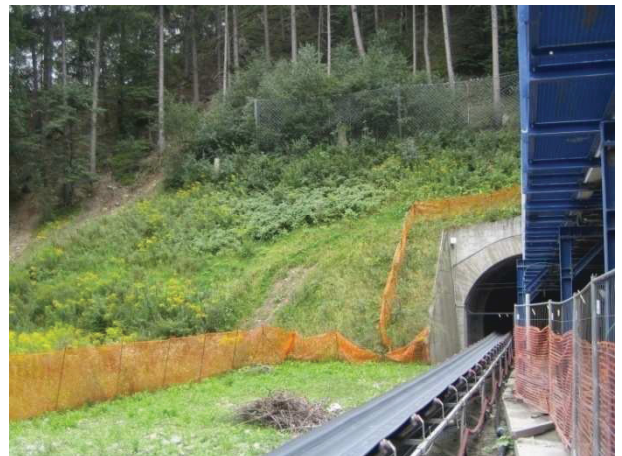
Portal Aicha- Hinterrigger Portale Aica-Hinterrigger
