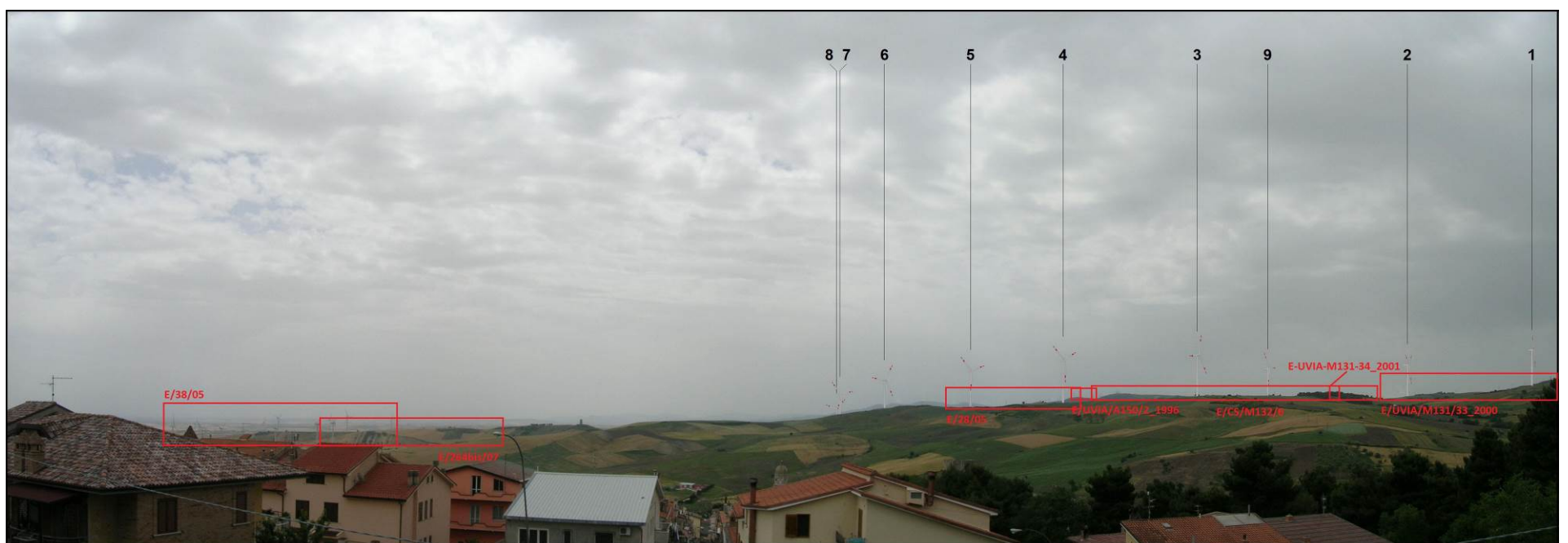
Vista 3b post operam
