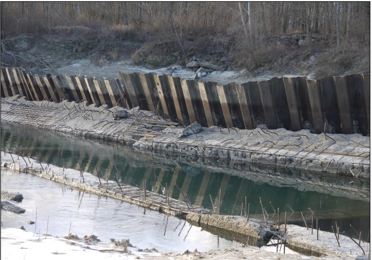
**FIGURA 11 – TRAVERSA (OPERE IN ALVEO) – DETTAGLIO PALANCOLATURA**
