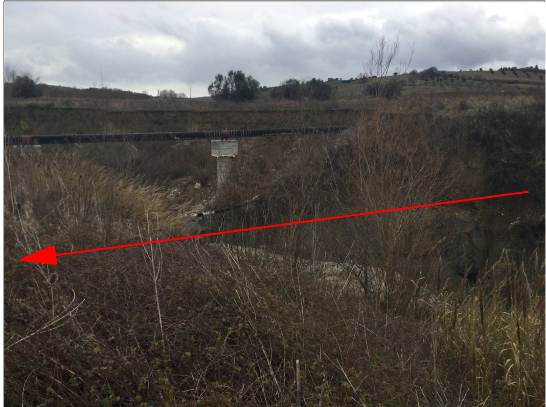
Attraversamento Trenchless (TOC Stampalone)
