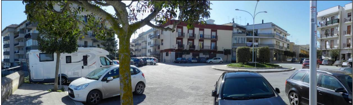
Vista 2_3 post operam
