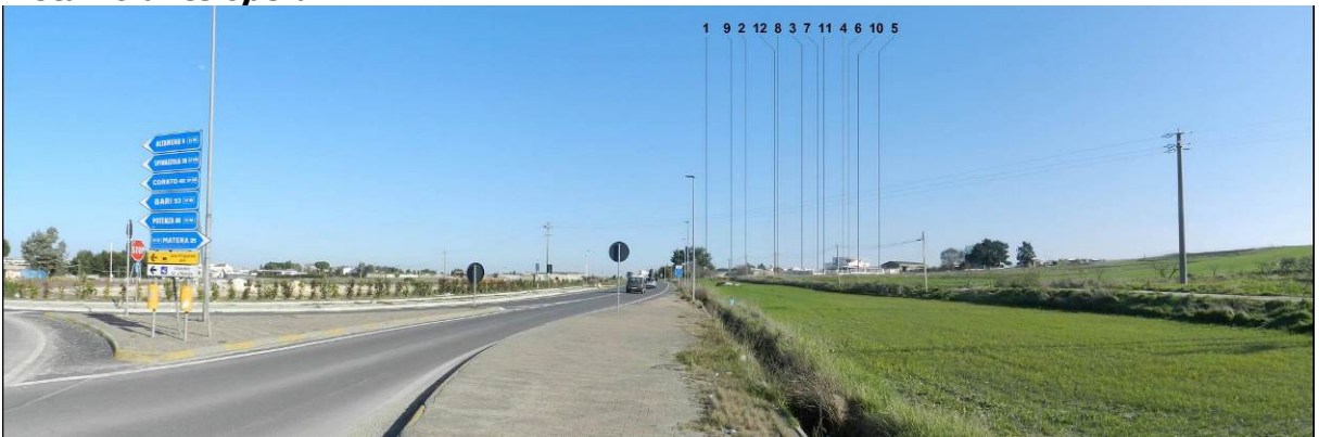
Vista 10 post operam
