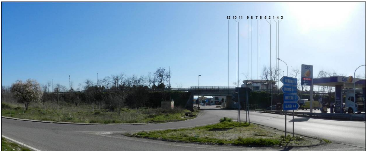
Vista 2_2 post operam
