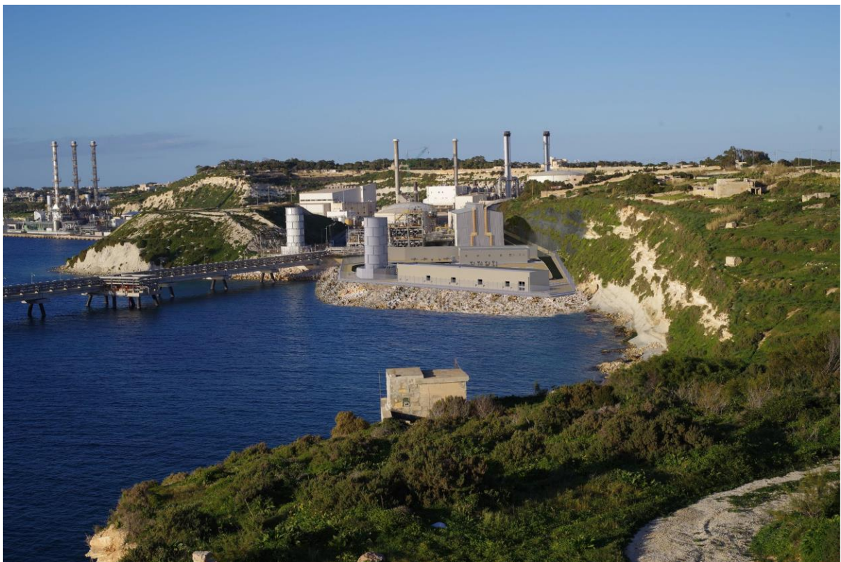
Figure 9: Viewpoint 1 - Photomontage of Scheme as seen from Carpark overlooking Delimara Power Station (Source: EIA Report [May 2021])
