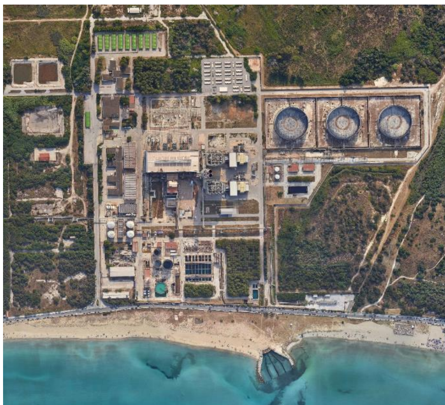
Figura 4.7.26 – Vista zenitale– Post operam
