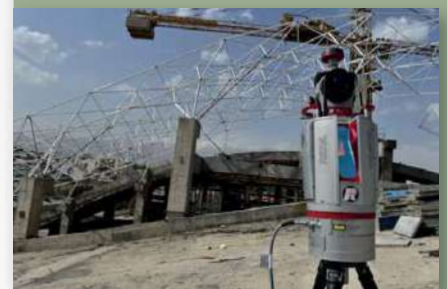
construction site monitoring
