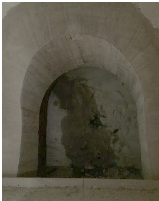
Foto 3 – Galleria Guinza - By pass pedonale
