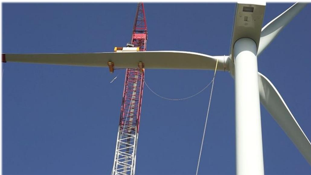
Figure 3: Wind turbine generator assembly
