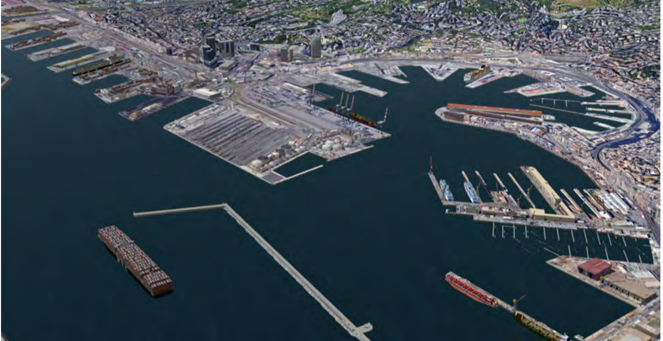
Figure 3.4: Aerial view of Solution 2
