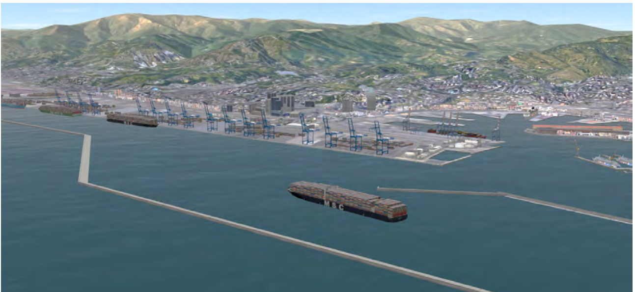
Figure 3.5: Aerial view of Solution 3
