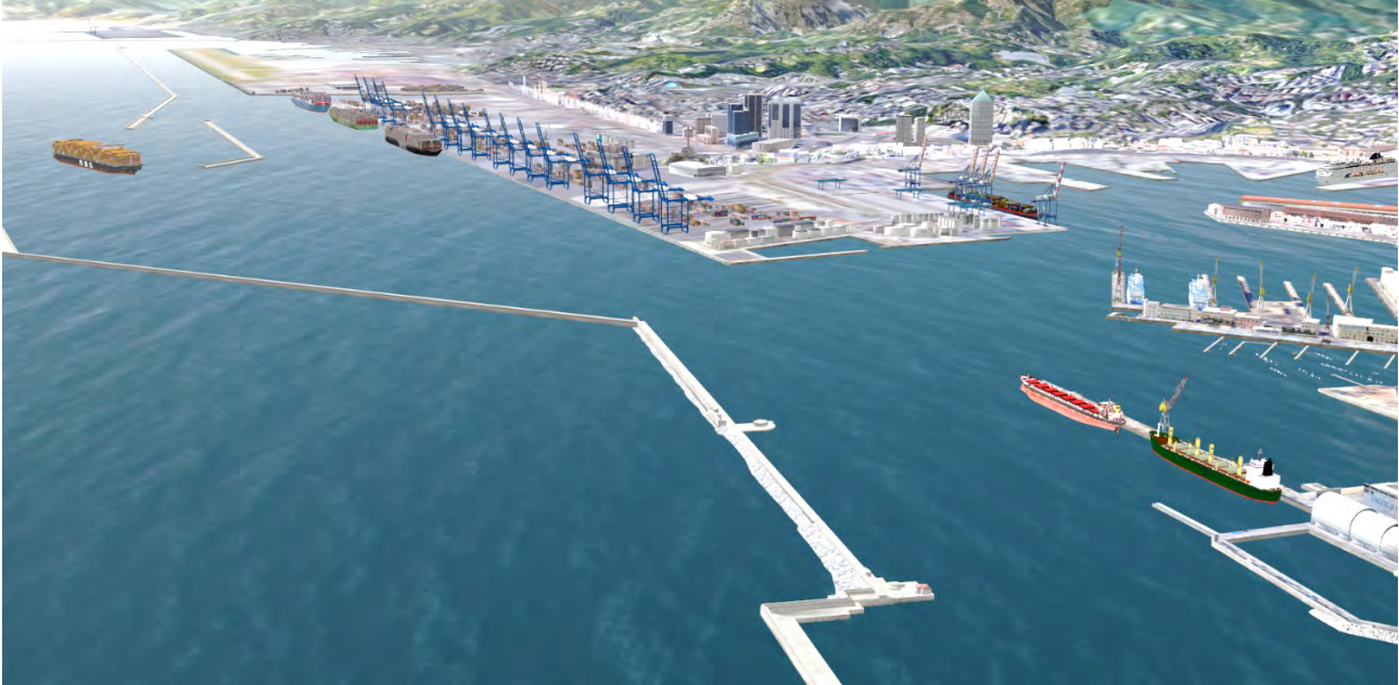
Figure 3.6: Aerial view of Solution 4
