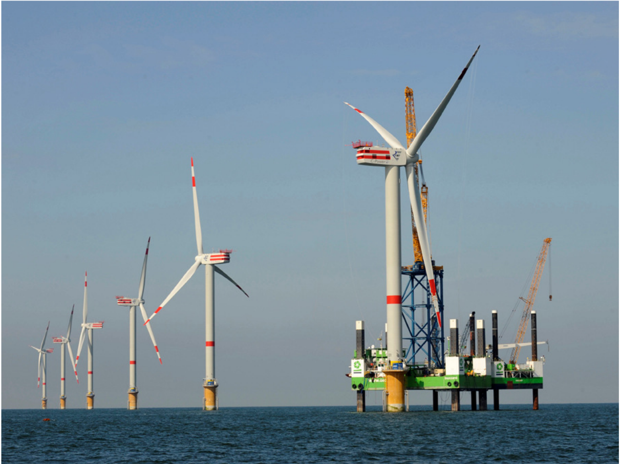
Figura B 7-6 6 aerogeneratori REpower 5M (P = 5 MW) assemblati - Thorntonbank wind farm [ http://www.repower.de ]
