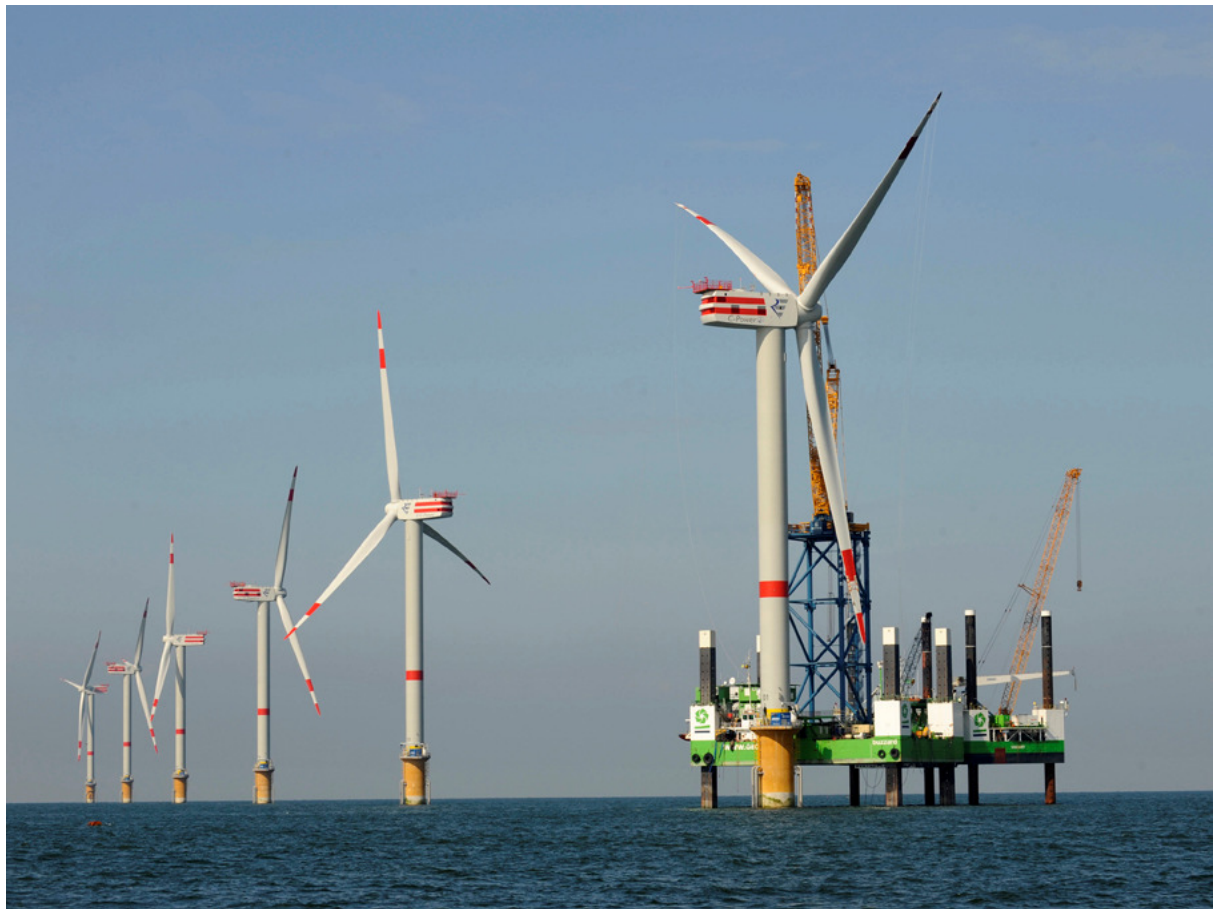
Figura 2-7 6 aerogeneratori REpower 5M (P = 5 MW) assemblati - Thorntonbank wind farm http://www.repower.de
