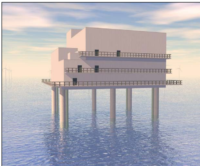
Figura 2-10 Electric Service Platform offshore
